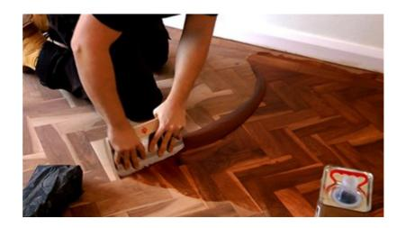
Water-based fillers need to be left overnight to dry, whereas solvent-based (for those from the US I think you would call it oil-based) fillers can be dry enough to sand off after 30 minutes if left in a room with good air circulation. The only problem with solvent fillers is that they aren't quite as flexible as water-based fillers.
