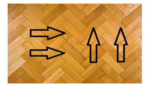
Next, you should switch direction from straight to across. This helps to eliminate any imperfections caused by the sander. This is especially true for people using hire tools as they
